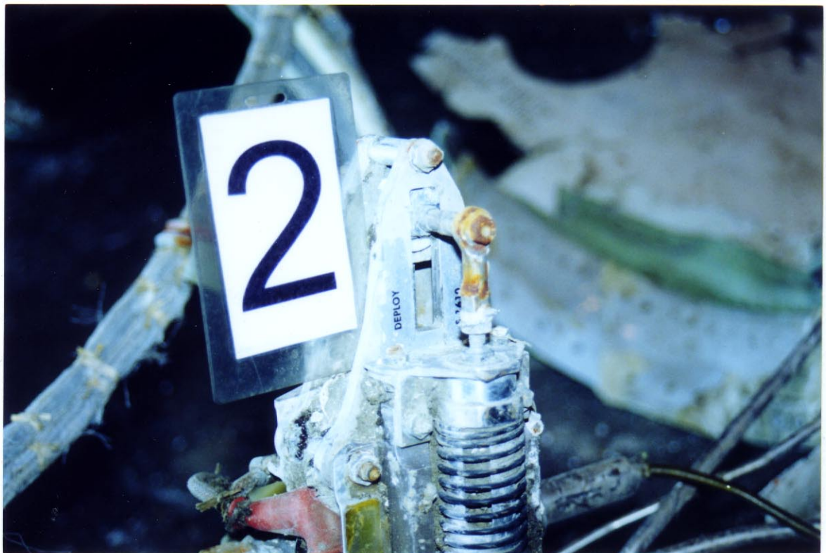
Photo 29. Closeup of No. 2 engine thrust reverser actuator showing indicator pin in reverser-stowed position.
