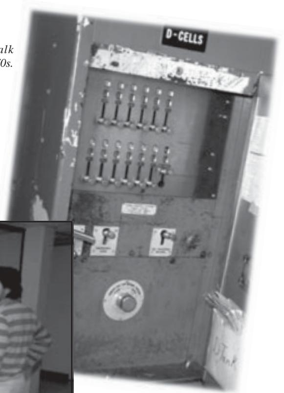
(Above) Control panel "D" Cells. (Note the hand crank to gang release all cells.)
