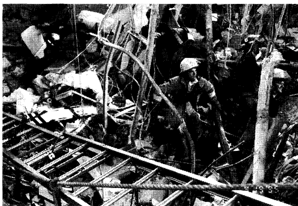
Members of OCFD Station 5 work to locate and remove the injured and dead in what will soon be known as the "Pit" area — the second floor day care. The area was a mixture of concrete, steel, office furniture, and other building contents. The ladder was used as a makeshift ramp to hand people up to rescuers so that the injured could be removed to the south side of the Murrah Building to a large triage area established in the plaza.
