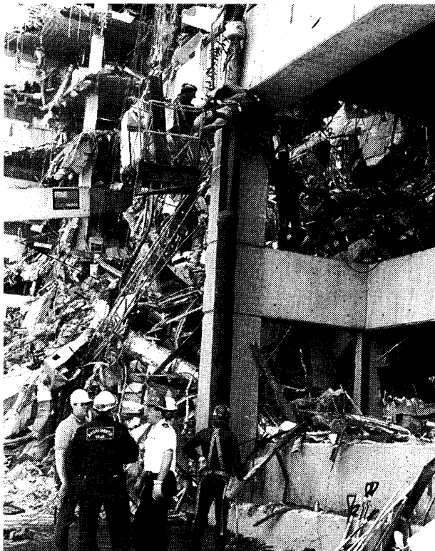
Construction workers erected this steel pipe reinforcement for column G12. Above the column is the remaining portion of the transfer beam, which had supported floors 3-9.
