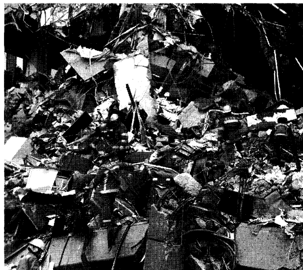
OCFD crews search the three-story debris pile at the east end of the Murrah Building. The officer is standing on the large concrete beam that spanned the building's length, supporting floors three through nine.
