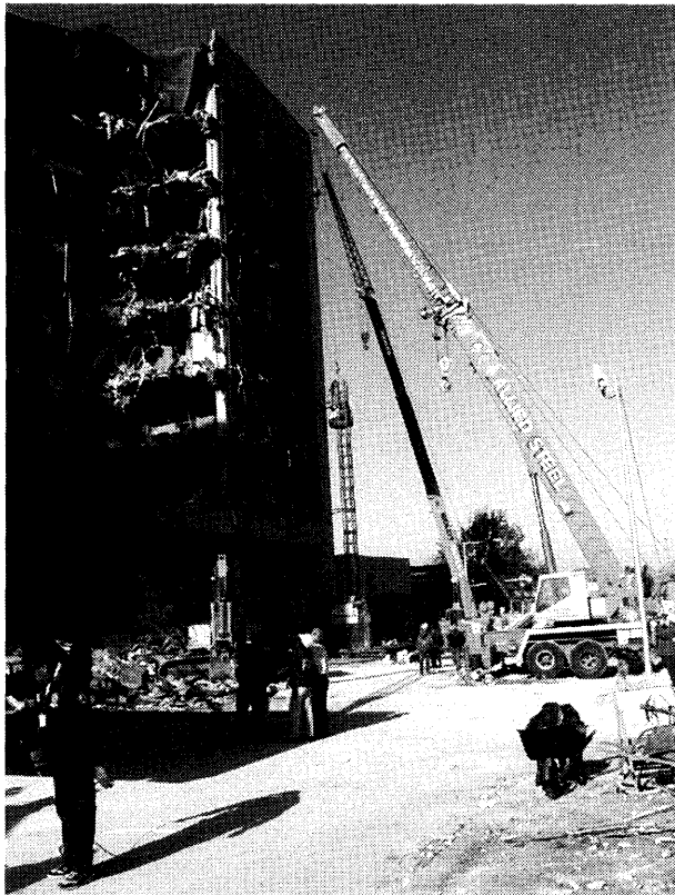
Cranes from Boldt Construction and Allied Steel work to place the manlift (elevator) to provide crews access to upper floors.
