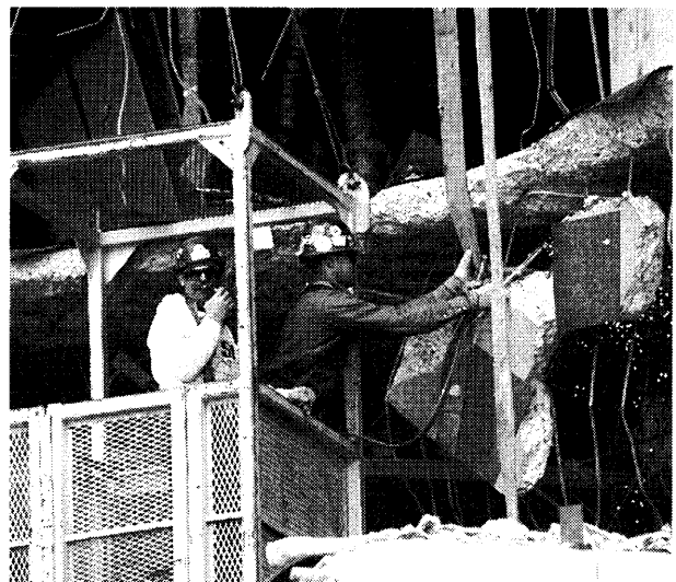
Steel workers operate from a lift hoisted by a crane and use a cutting torch to remove smaller, but deadly, "widow makers" hanging over the edge and above the heads of rescuers below.
